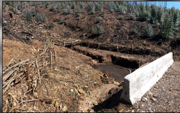
detention basin (combating soil erosion)
